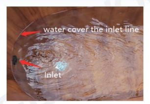
(4) Use a water hose to inject water DIRECTLY into the tub water inlet. Bubbles will be flushed out from the tub water outlet. This procedure will remove any air stuck in the chiller system.
