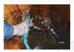
(5) Keep injecting water DIRECTLY into the tub water inlet until no more bubbles are coming out from the water outlet. This may take 2-3 minutes. When done, please remove the hose.
