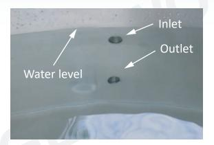
4 Use a water hose to inject water DIRECTLY into the tub water inlet. Bubbles will be flushed out from the tub water outlet. This procedure will remove any air stuck in the chiller system.
