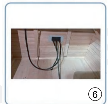
Step 6: Install Plug
