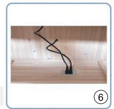
Step 6: Install Plug(Leg+ Foot Heating)
