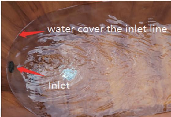
④ Use a water hose to inject water DIRECTLY into the tub water inlet. Bubbles will be flushed out from the tub water outlet. This procedure will remove any air stuck in the chiller system.
